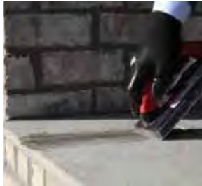
PIC 1. Fill joint with grout.
