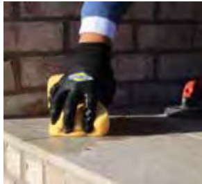
PIC 2. Remove excess grout with clean water.
