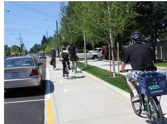
The separated bike lane shown above is protected from motor vehicle traffic through on-street parking and is commonly known as a "parking-protected bike lane."
