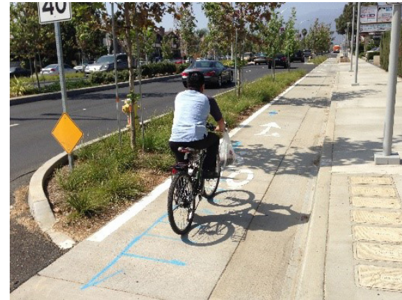
The separated bike lane shown above is separated from motor vehicle traffic by a concrete curb and landscaping.
