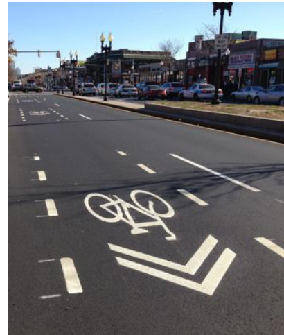
Super sharrows can either have dotted line markings, above left, and/or be enhanced with green paint, above right.
