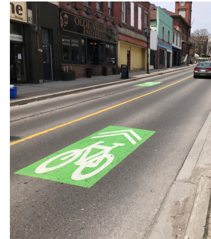
Super sharrows can either have dotted line markings, above left, and/or be enhanced with green paint, above right.
