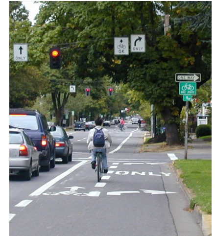
Two stage turn queue boxes, above left, provide a dedicated space for bicyclists to turn left, often when crossing multiple lanes of traffic. A combined bike lane / turn lane, above right, can improve positioning for motor vehicles and bicyclists at right turns.
