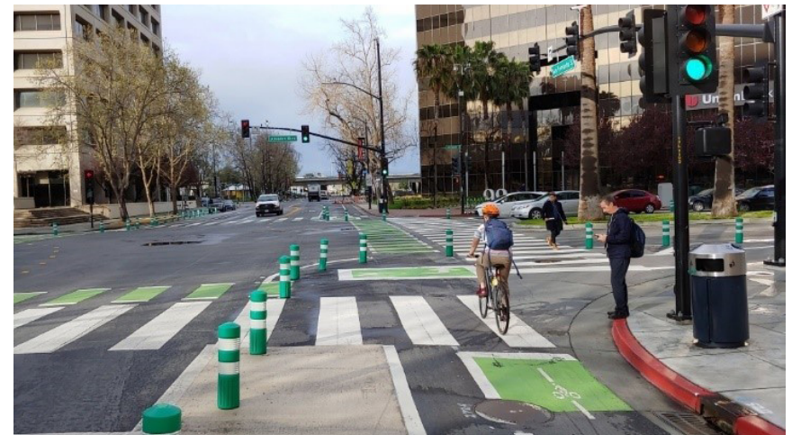
The photo above shows a protected intersection using low cost materials such as plastic bollards and paint.
