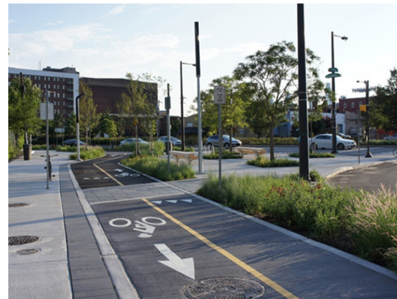
The separated bike lane shown above incorporates landscaping into the buffer.
