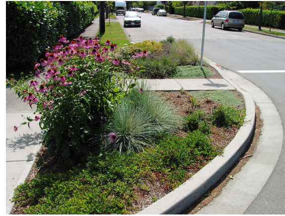
The curb extension shown above can be incorporated into the long term design of neighborways to beautify the street, reduce stormwater runoff, and slow down motor vehicles.
