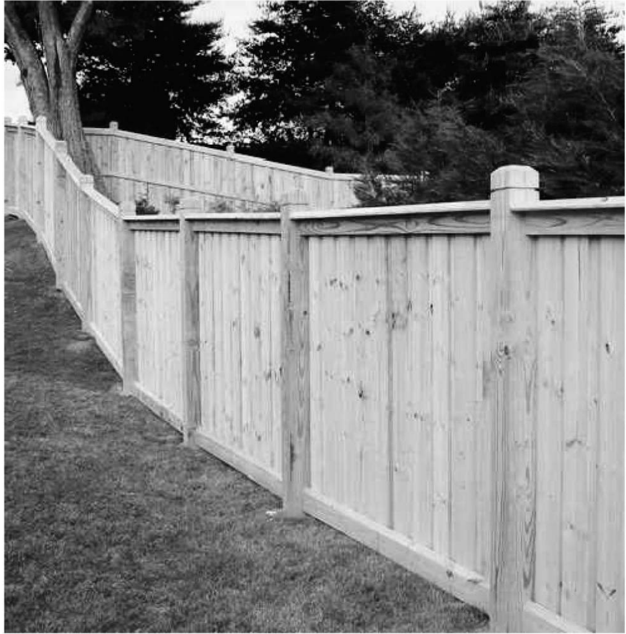
7' Board on Board Privacy Fence Detail
