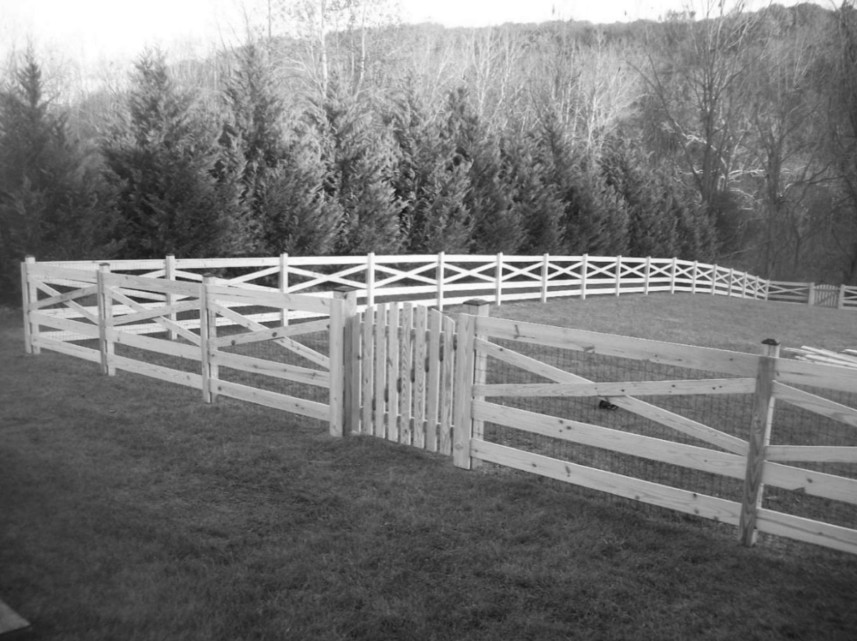
5' Rail and Crossbuck Board Fence with Wire Mesh Detail
