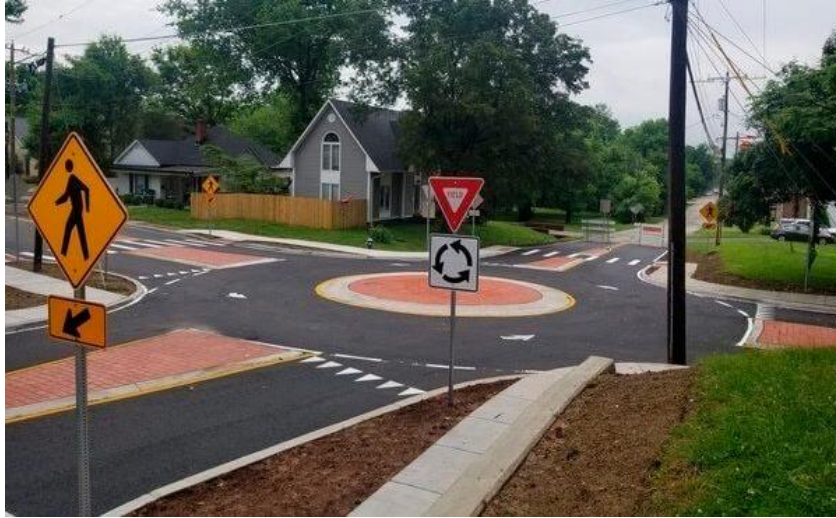
Figure 13. Example of a Mini-Roundabout in Hardin County, KY (Source: Times-Tribune)
