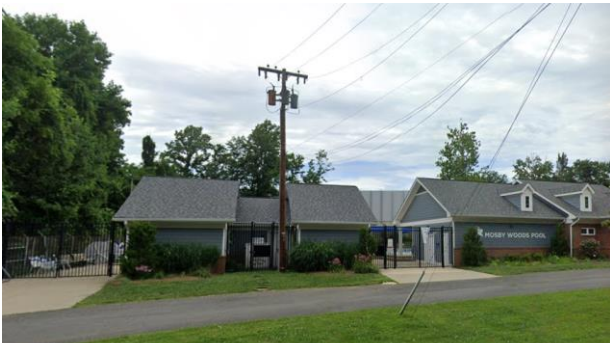
Mosby Woods Pool fronting Fair Woods Parkway at Blue Coat Drive. Source: Google Earth.
