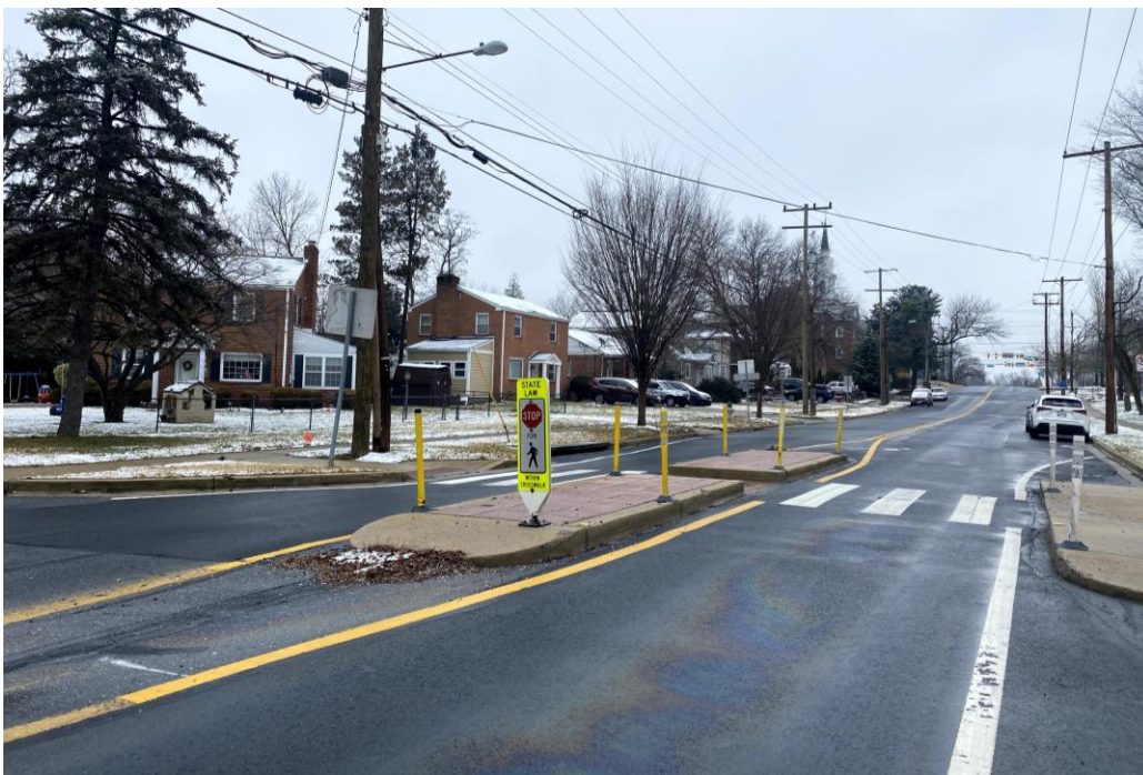
Figure 15. Example of a Spot Median Island
