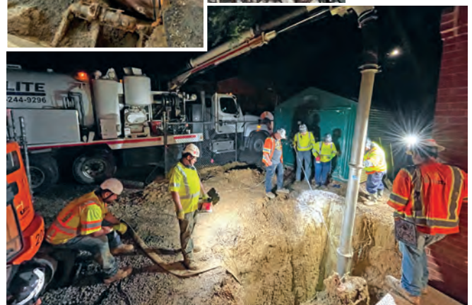
ABOVE: A vacuum truck removes wet sediment from the excavation site.
